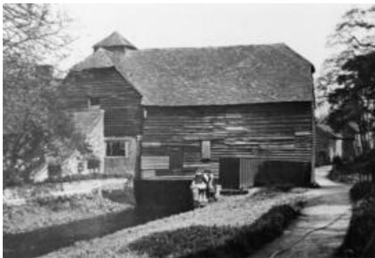
Weydon Mill was thought to be first used to mill flax before it milled corn. The undershot water wheel was turned by the mill race which you can still see. The mill was producing food for the local populace until about 1912 when it ceased working after more than 800 years of public service. It was finally demolished in 1919. In about 1955 a bungalow was then built on the site, later extended and upgraded in 1991/2 into the present bungalow.
